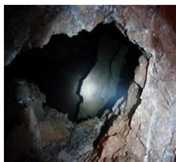
图5 溶洞揭露照片 Fig.5 Photo of displaying karst cave
